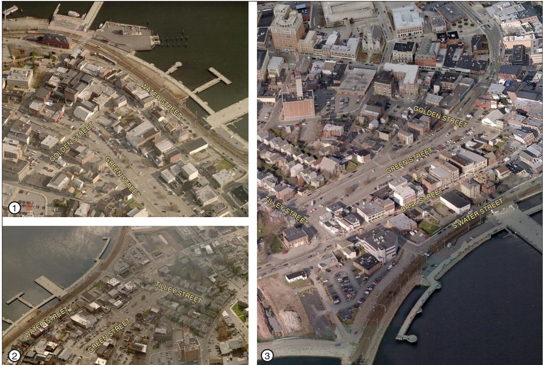
FIGURE 13: PHOTO INVENTORY – AERIAL VIEWS OF PROJECT AREA
